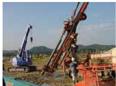
斜杭削孔状況 =15°
